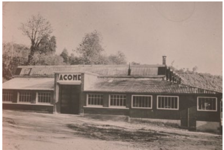
ACOME's 1 st site in Normandy (Usine des Vallées, Mortain) sold to the community in 2021.
