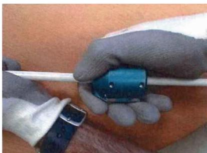
Figure 1 : opening a CU cable
