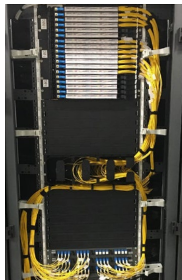
Horizontal management subrack 3U fitted in a 19" frame
