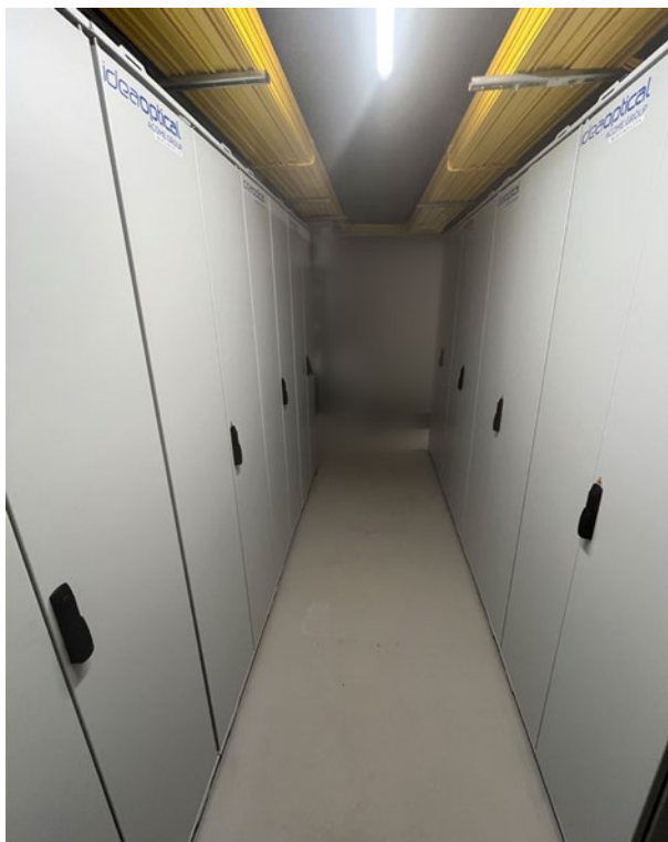
Installation of Optic-Run in the Meet-Me-Room
